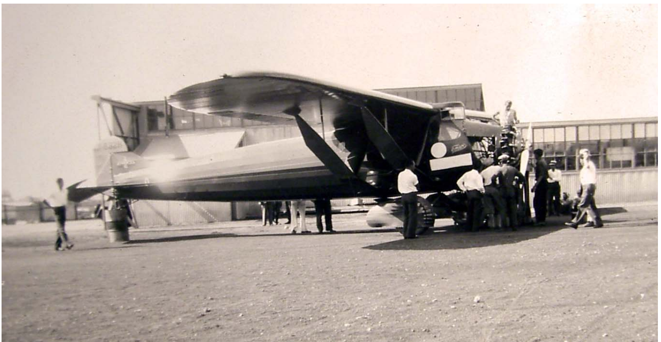
The second EMSCO aircraft (X-832H) was the first of the B-3 series, seen here readying for a test flight at Long Beach. In lower photo, note glare reflecting off immaculate finish for which EMSCO aircraft were famous. Russ Gerow's note on this picture reads: "Jack Reid's 'Death Ship.' This ship lifted over 6,000 lbs gas and oil with a single 300 h.p. engine. Flown by Reid and Bronte at Long Beach Airport. Reid was killed in ship at Cleveland. Emsco aircraft designed by Chas. Rocheville." Reid, an EMSCO employee and old Navy friend of Rocheville, set a new world's solo endurance record with this aircraft on Aug. 21, 1929, but fell asleep and crashed 38 hours 40 minutes into the flight. In a snafu emblematic of EMSCO's chronic hard luck, Reid was actually airborne hours earlier waiting for the delayed official timing of the flight to begin. Photo Russ Gerow, Long Beach Airport, 1929. Russell T. Gerow Collection
